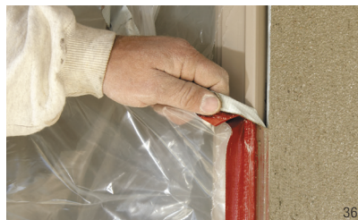
Strong backing of 3M™ Outdoor Masking and Stucco Tape 5959 pulls through stucco, EIFS and other heavy coatings in one piece.
